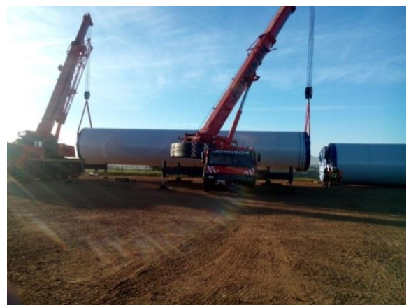
Figure 3-8: Transportation of a Tower section
