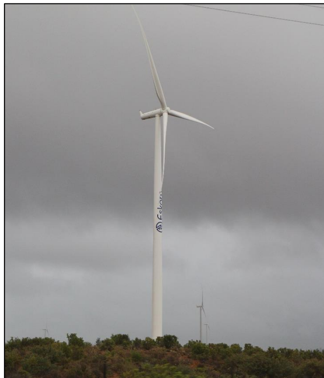
Figure 7-18: Markings on the tower (or nacelle / blades) increase the visual intrusion of the turbine
